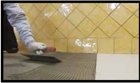
Fig.28 - This method refers only to adhesives that bear the indication "single-layer" by the manufacturer. Spread adhesive on the complete surface of the support. Follow the instructions of the manufacturer of the adhesive as regards type of spatula and spreading methods.
