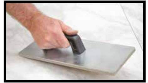
Fig.30 - After laying the tile, make sure it is firmly bound to the underlying surface to prevent gaps and air bubbles forming. For this purpose you must use a tile beater with a rubber bottom (for example Raimondi "142G").
